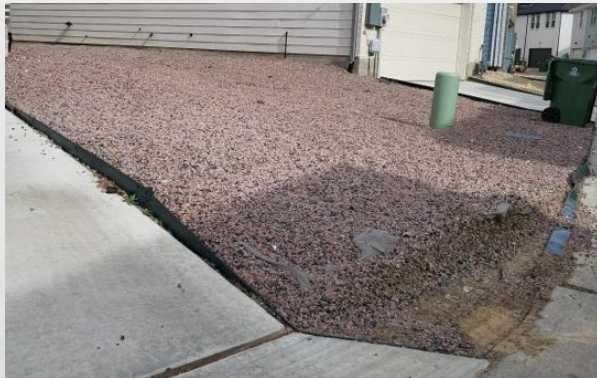
Repairs to alleyways
